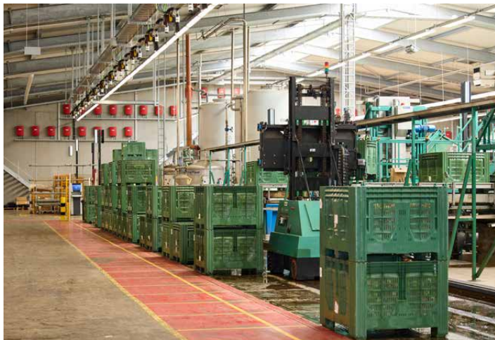
A transverse transfer car (Binmatic, front right) picks up the bins containing the sorted apples and stacks them on the opposite side to be collected by the high-lift truck drivers.
